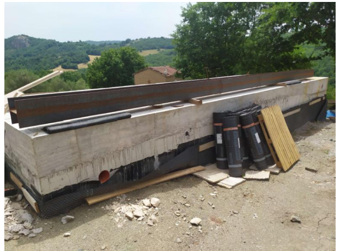
Rainwater collection tanks
