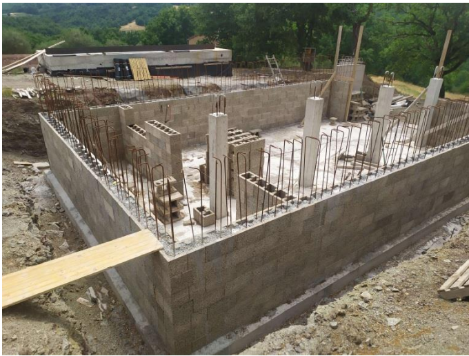
Foundations and basement wall
